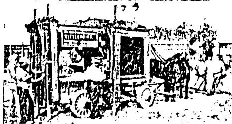
Curtis Multiple Stake Driver Powered with a 8 H. P. WITTE Engine.
